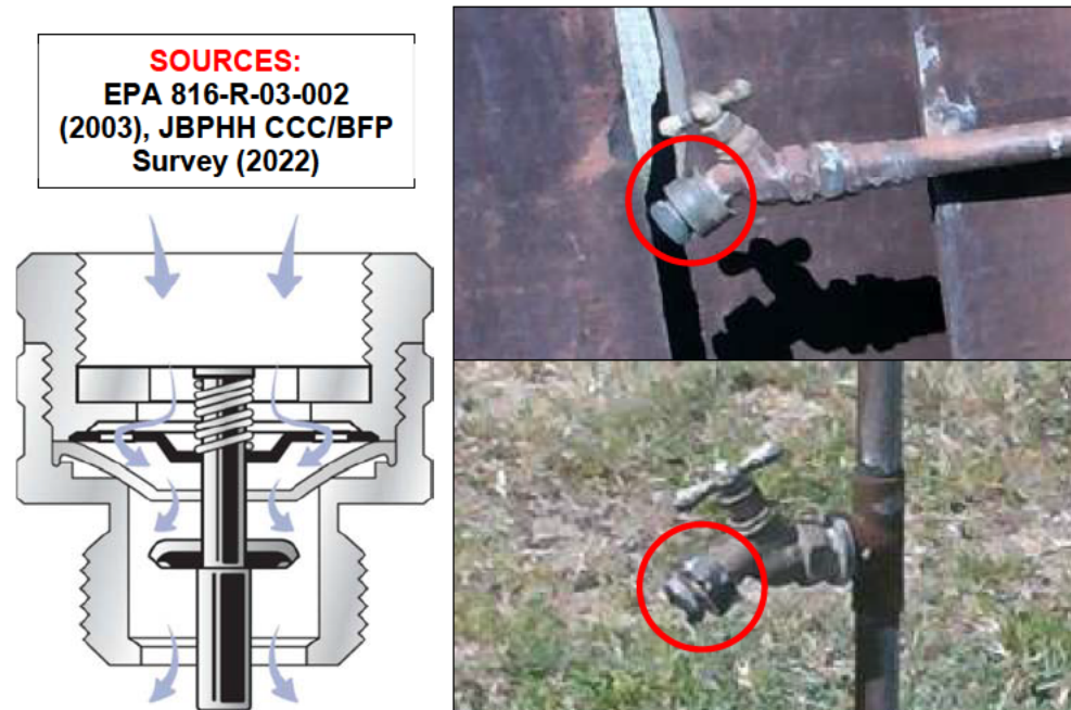
Figure 3-3 Hose Bibb Vacuum Breaker Examples
