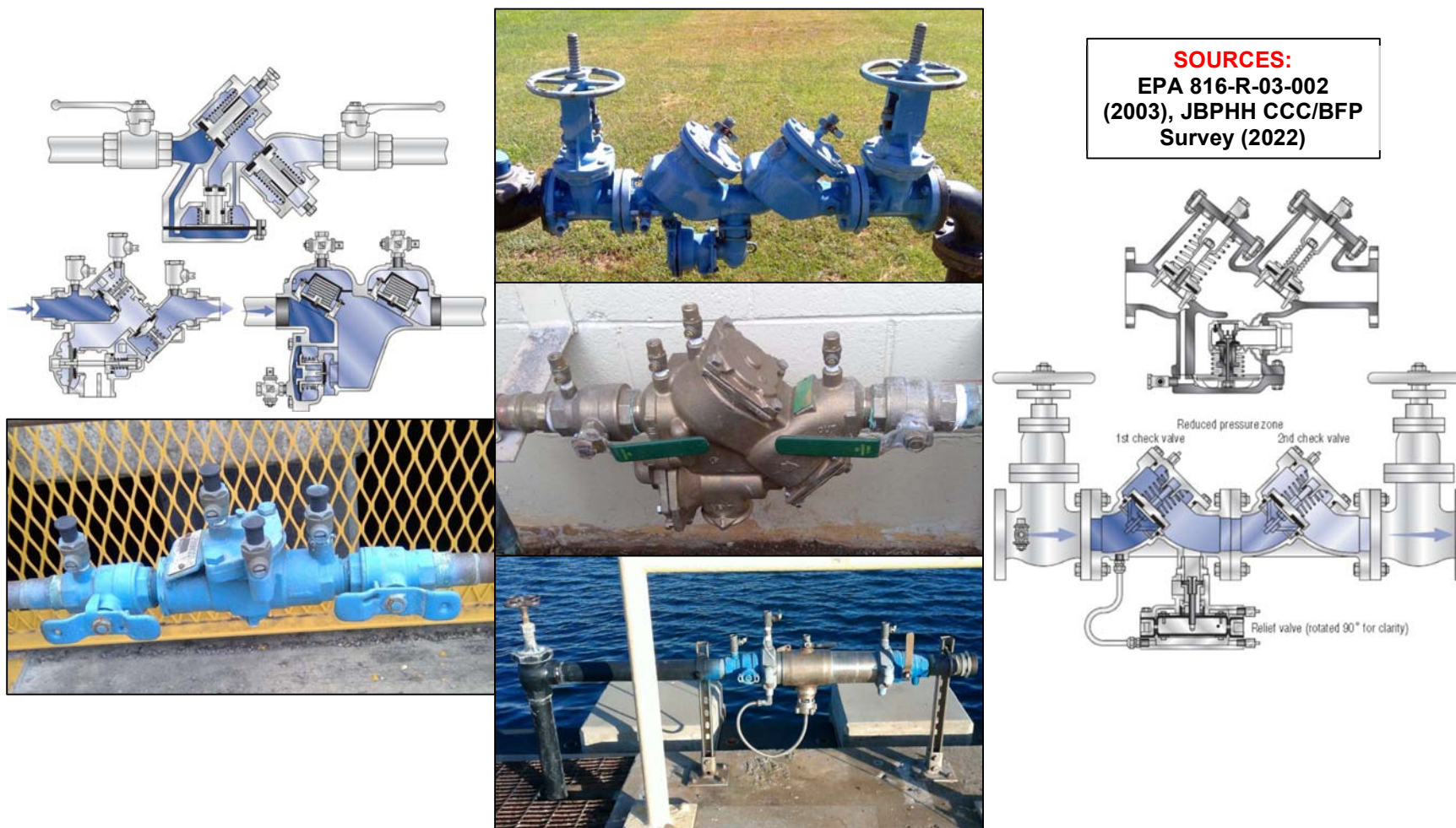
Figure 3-4 Reduced Pressure Zone (or Principle) Assembly Examples
